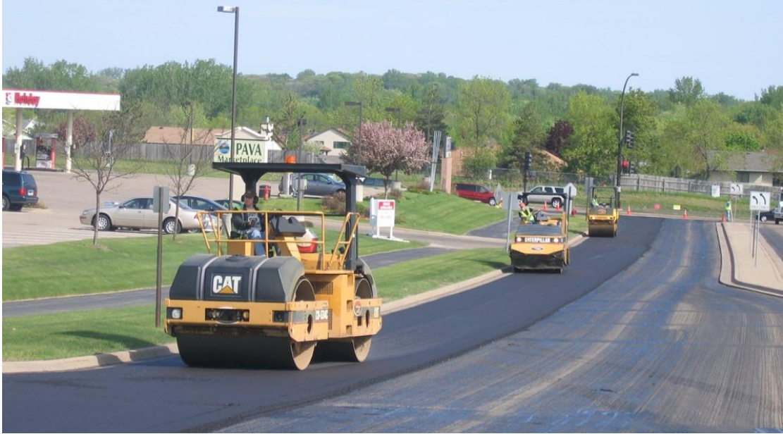
Grind and Overlay
