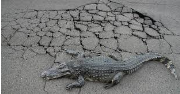
Alligator Cracking
