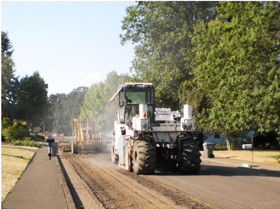
Full Depth Reclamation
