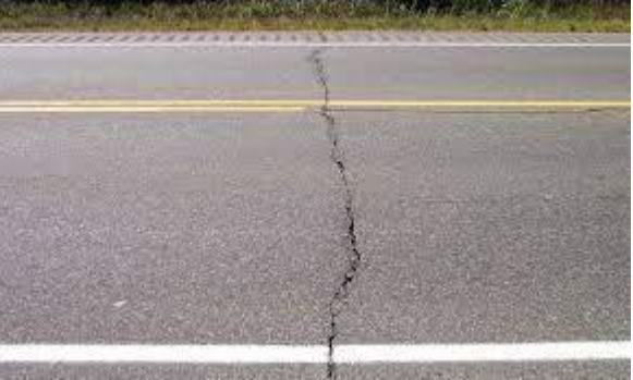
Transverse Cracking
