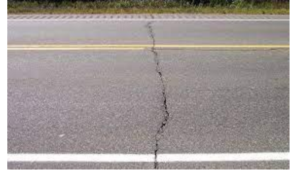
Transverse Cracking
