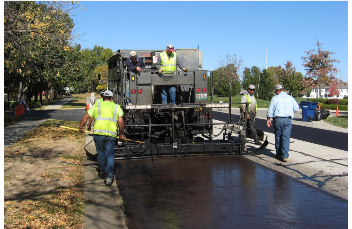
Slurry Seal
