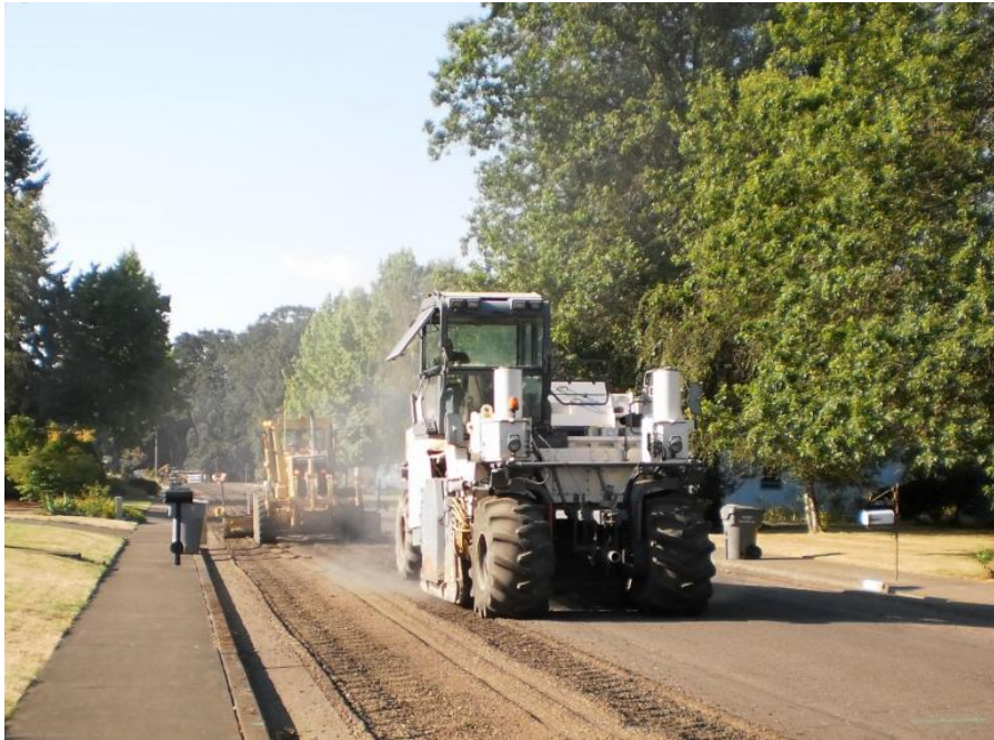
Full Depth Reclamation
