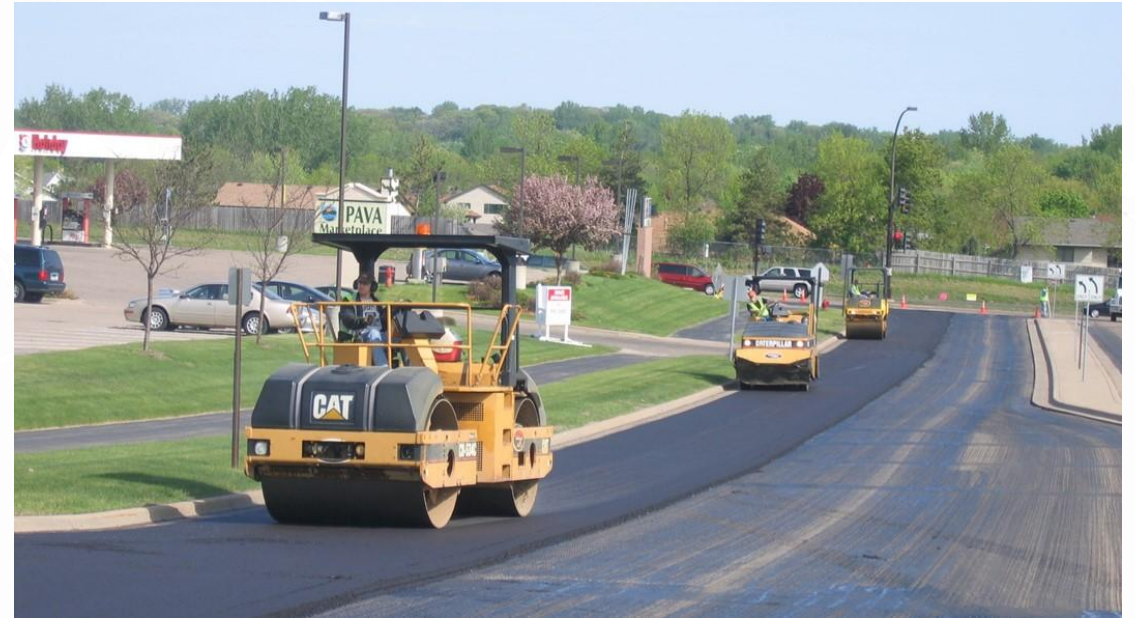
Grind and Overlay
