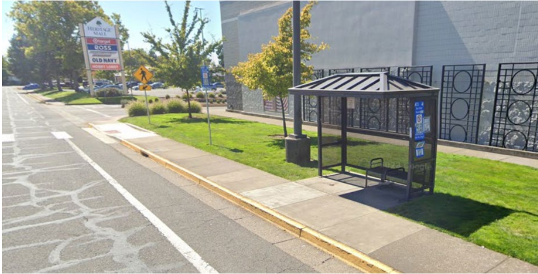
Figure 2 Shelter and Pedestrian Cross at Heritage Mall Clay Street Stop
