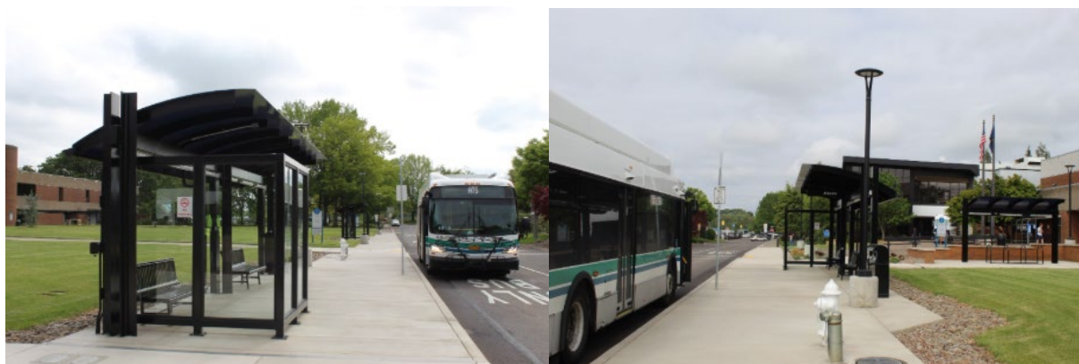
Figure 2-1 & 2-2 ATS Boarding at Second Bus Shelter
