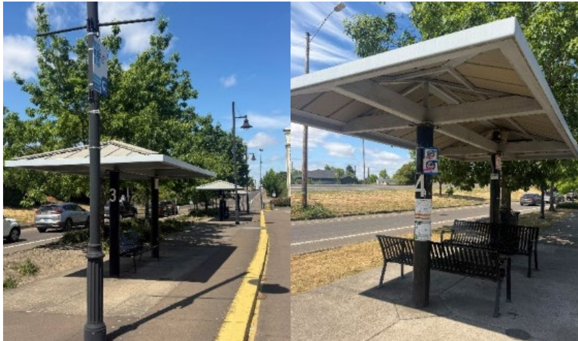
Figure 7-1, 7-2 & 7-3 Albany Amtrak Station Numbered Shelters
