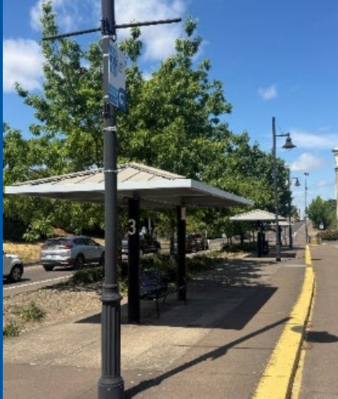
Shelter #3: BAT Signage
