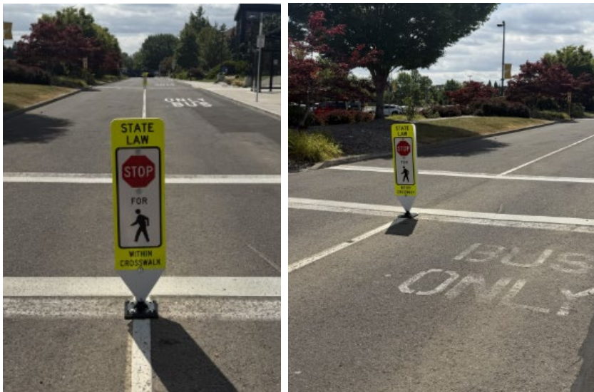
Figure 5-1 & 5-2 Pavement-Embedded Signage at LBCC
