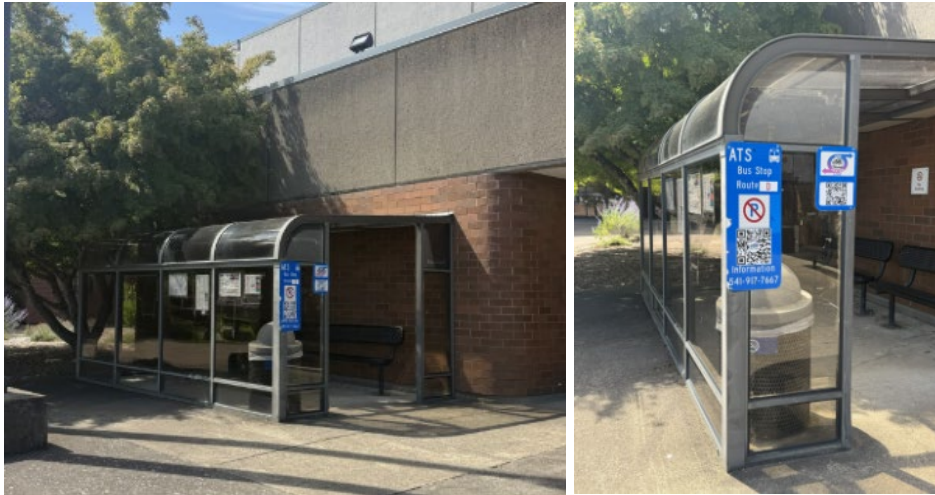
Figure 1-1 & 4-2 Bus Shelter Attached to LBCC Building
